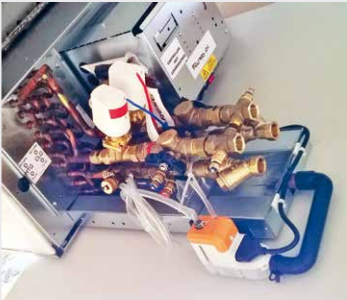
All Dunham-Bush fan coils are available with optional extended drip tray and fitted condensate pumps
