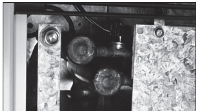
Type 1 LTC and manual air vent
