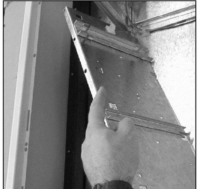
Diagram 4 : Fan and inner side plate removed
