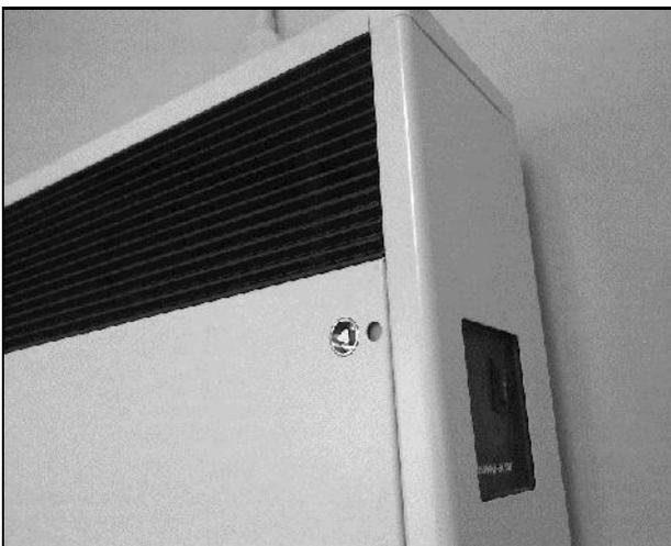
Diagram 10: Lock indicator green - panel locked
