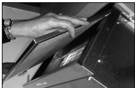
Diagram 13: Withdraw the filter
