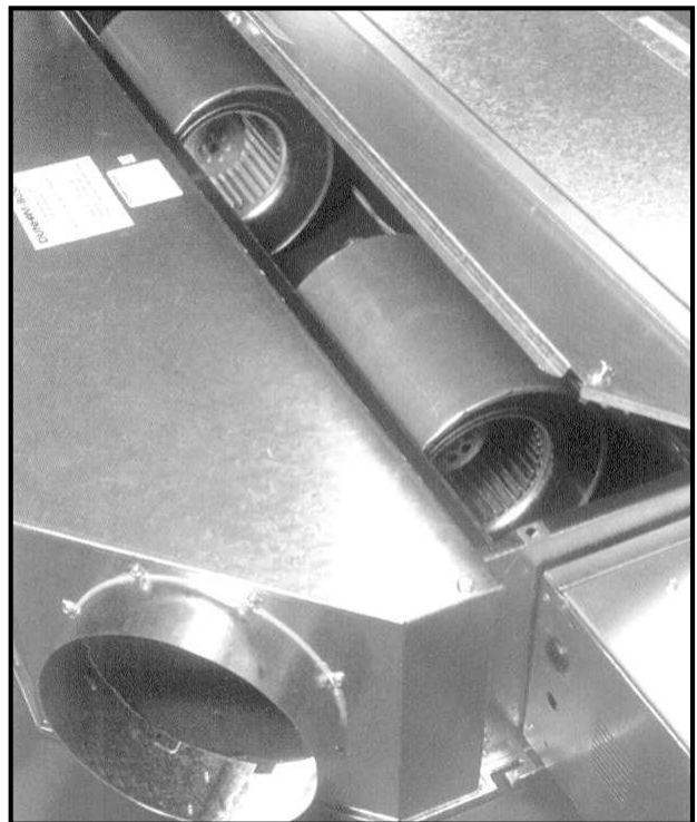
Diagram 6: Fan access panel
