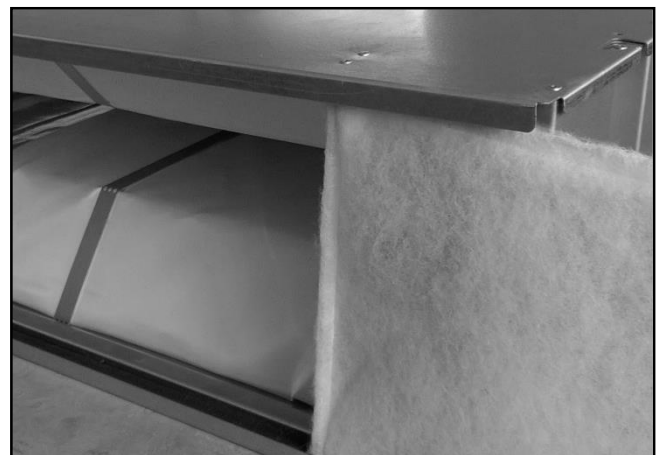
Diagram 9: Suspend attenuator with drop rods through suspension slots; adjust suspension to mate attenuator to unit inlet. Refit air filter to attenuator inlet.
