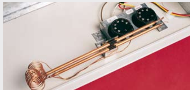
Image 2: Fitted of/off and speed change thermostats
