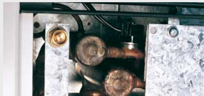
Image 3: Fitted type 1 low-limit thermostats
