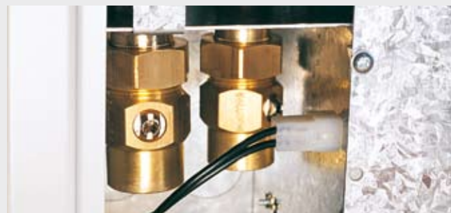
Image 5: Fitted isolating valves - model SA only
