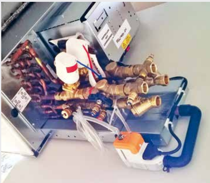
Optional extended drip tray and fitted condensate pump
