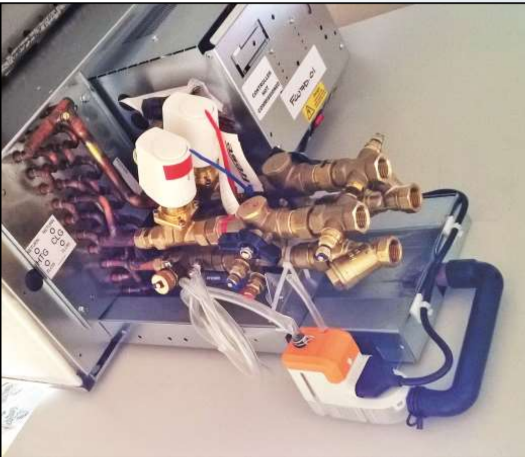
Optional extended drip tray with control valve assembly fitted condensate pump
